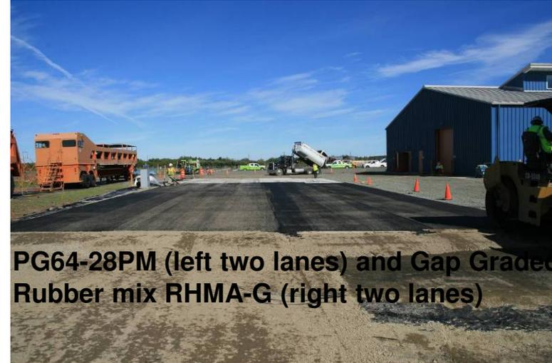
**PG64-28PM (left two lanes) and Gap Graded Rubber mix RHMA-G (right two lanes)**
